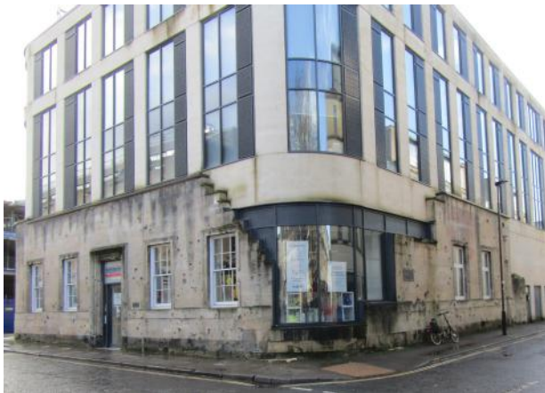
Fig. 1: The former Labour Exchange building, built 1938, repaired 2017, James Street West, Bath, with shrapnel damage in the lower few metres.
