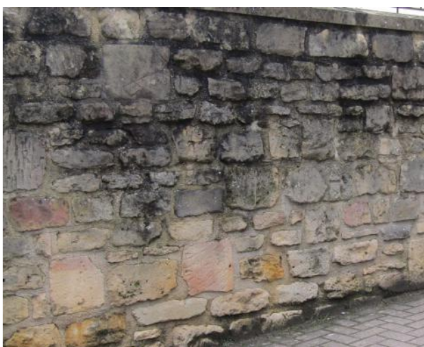
Fig. 11: Blocks of pink Bath Stone in a wall by Julian Road, likely coming from a nearby building which suffered fire damage.
