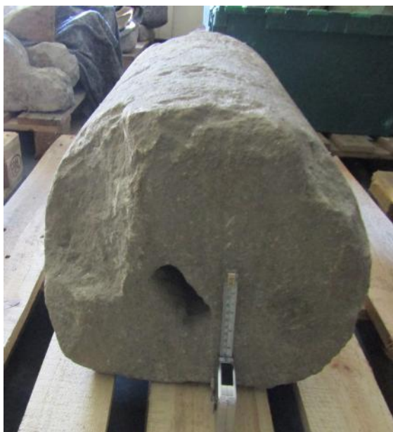
Fig. 5: Lewis bolt hole in one end of a Roman column of Bath Stone; length of bolt hole 9 cm. Stone store, Bath.
