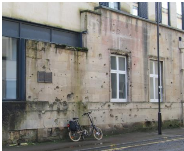
Fig. 2: The Labour Exchange, Milk Street side, with bomb damage and pink stone upper right from the effects of fire on higher floors.
