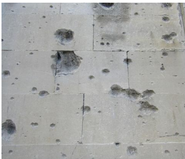
Fig. 3: Labour Exchange impacts marks, variable size. Size of stone blocks 30 cm high.
