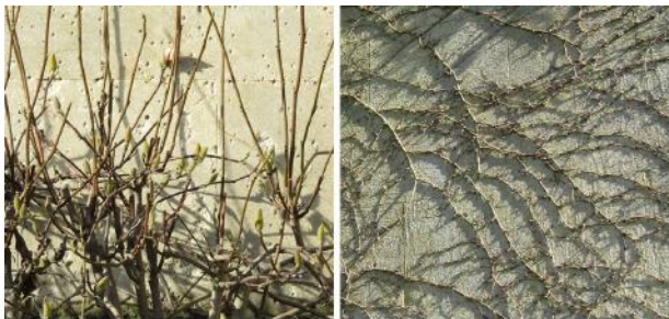
Fig. 17: Vegetation growing against/on the front walls of buildings, magnolia in the Royal Crescent with small impact holes behind and Virginia creeper in Queen Square.
