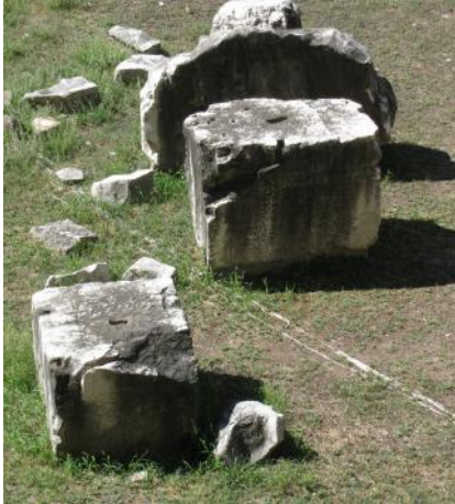
Fig. 2 A: Two stone blocks near the Forum, Rome, with bolt holes (approx. 10 cm in length).
