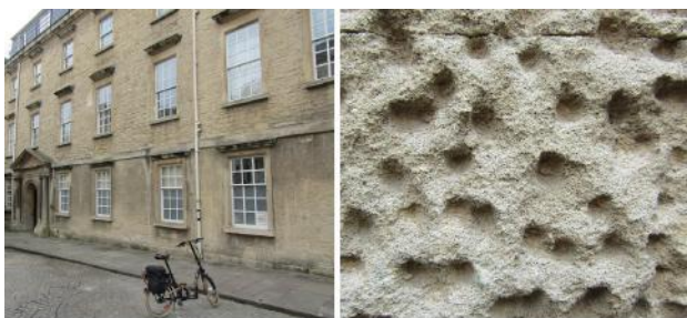
Fig. 19: Vermiculation on the wall of The Hospital of St John the Baptist.
