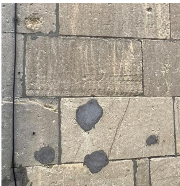
Fig. 8: Four cement-filled impact craters and one empty one higher up on the wall of a house in Third Avenue, Oldfield Park, in the immediate vicinity of a bomb site.
