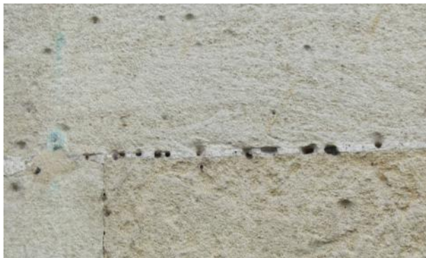
Fig. 21: Holes which could be from the activities of masonry bees. Or more nails for the clematis (or both)?
