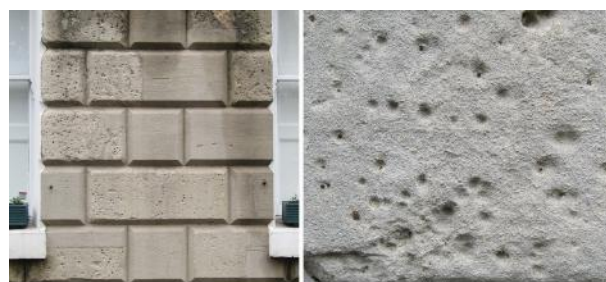
Fig. 13: A wall in Queen Square with some new stone but numerous small impact marks on older stone, with a range of features.
