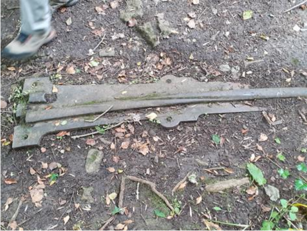
Fig. 5: Cast iron tram way lines
