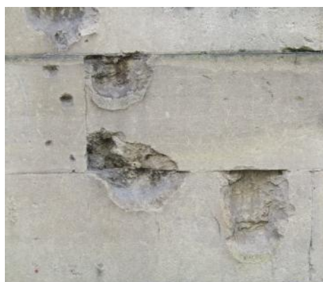
Fig. 5: Labour Exchange impact crater shape affected by stone block boundaries.
