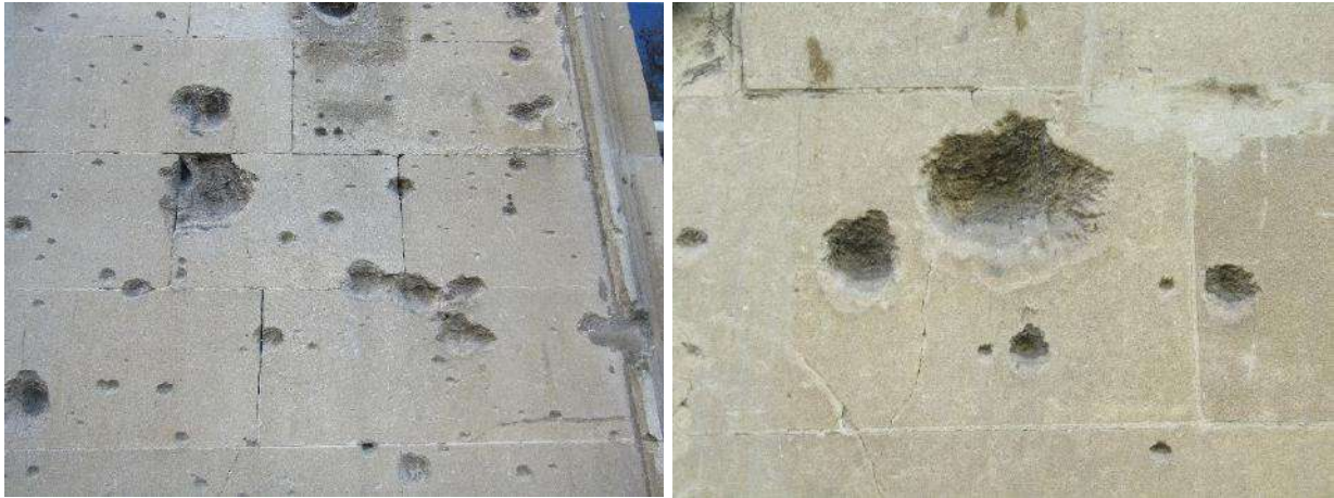
Figures 3 & 4. Range of sizes of impact marks; many are quite smooth inside. The stone blocks are 20 cm high.
