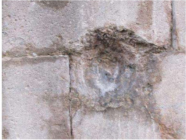
Figures 7 & 8. Impact craters across areas where 2 or 3 blocks are in contact with loss of the boundaries. Note the granular nature of the weathered surface of the limestone, contrasting with the finer-grained-looking surface of the stone within the crater.
