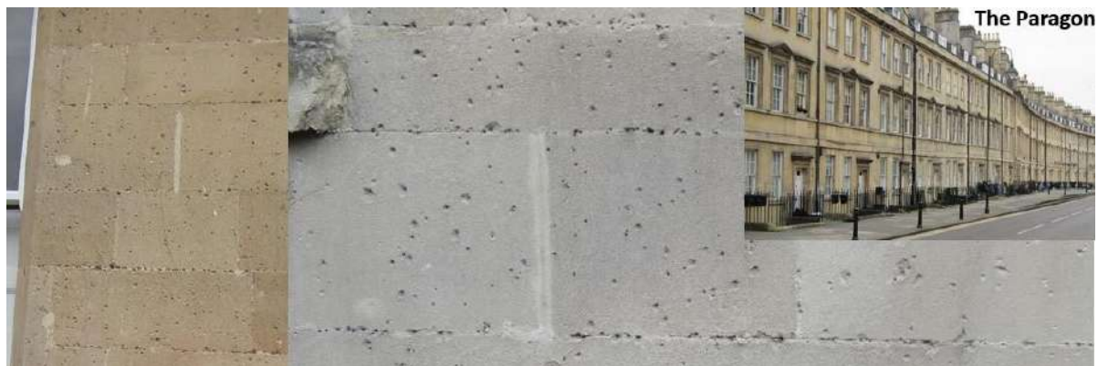
Figure 4. Small impact holes on a house in the Paragon; Bath Stone blocks 30 cm high.
