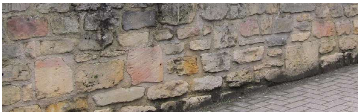
Figure 1. Pink-red Bath Stone blocks, likely resulting from fire damage, in a wall by Julian Road.
