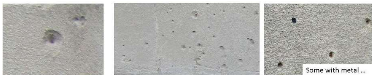
Figure 5. Details of small impact craters from the front walls of several houses in the Paragon.
