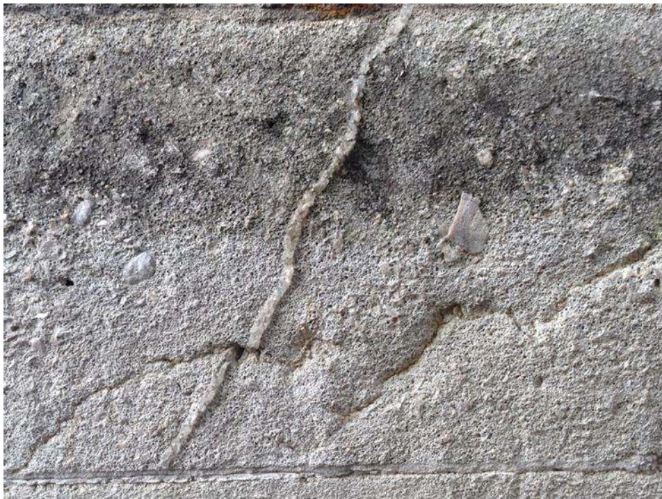
Figure 3. A subvertical fracture in shelly bioclastic Bath Stone filled with calcite, which is offset by a sub-horizontal stylolite, along which there is a thin insoluble residue (clay). Great Pulteney Street, Bath.
