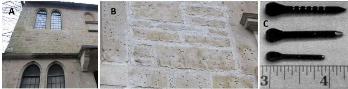
Figures 7A, 7B. Small impact craters on the front wall of Magdalen Hospital at first-floor level. 7C: Flechettes – aerial darts dropped by planes, are the right size for the small impact marks.
