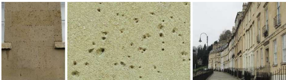
Figure 6. Small impact craters on front wall of a house at Walcot Parade.
