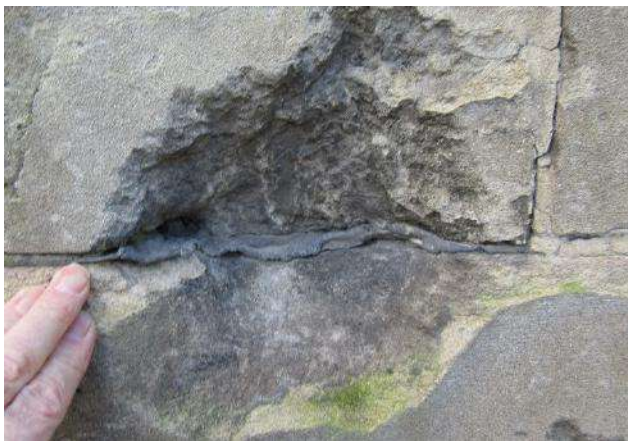
Figures 9 & 10. Deformation of the lead damp course where it occurs within an impact crater: lead is folded and contorted. Note finer-grained appearance of limestone inside the crater compared to outside on the weathered stone. The black colouration in Fig. 9 (and 6 and 7) is likely weathering and organic-microbial staining.
