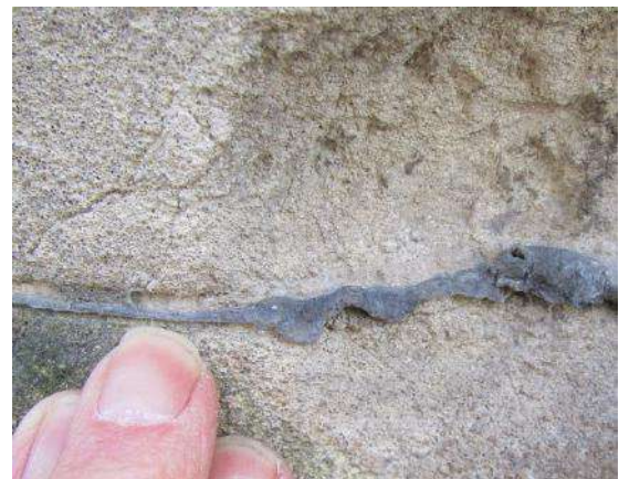
Figures 9 & 10. Deformation of the lead damp course where it occurs within an impact crater: lead is folded and contorted. Note finer-grained appearance of limestone inside the crater compared to outside on the weathered stone. The black colouration in Fig. 9 (and 6 and 7) is likely weathering and organic-microbial staining.
