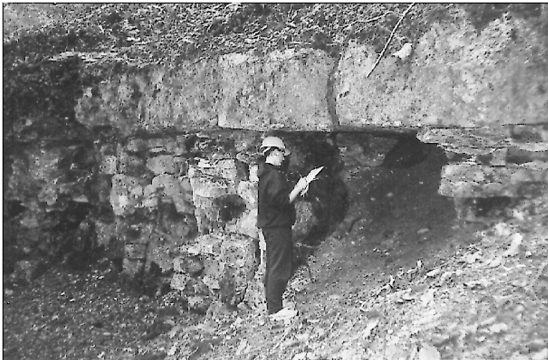
Victoria at Site One, Brown's Folly. The Roof Bed can be seen clearly above the Bath Oolite. This is an adit mine, the roof of which has collapsed (Photograph by Siobhan Moore)
