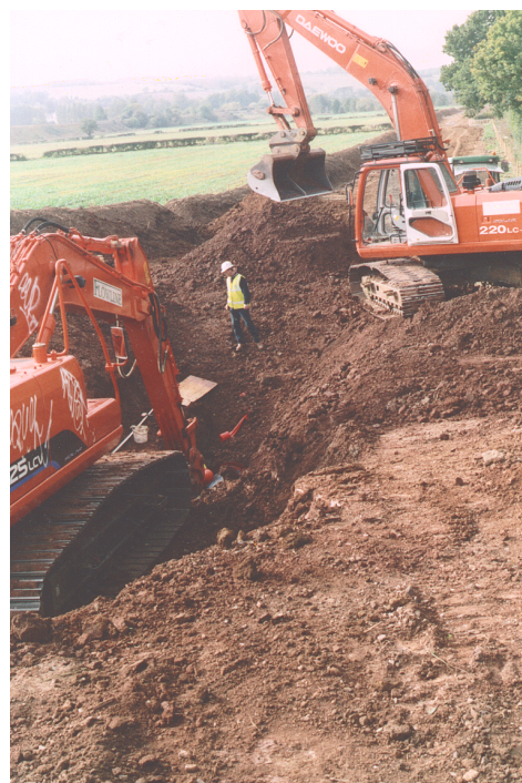
Photograph looking west towards Saltford. The pipe trench has been excavated and exposed fine river silts overlying Upper Triassic mudstones
