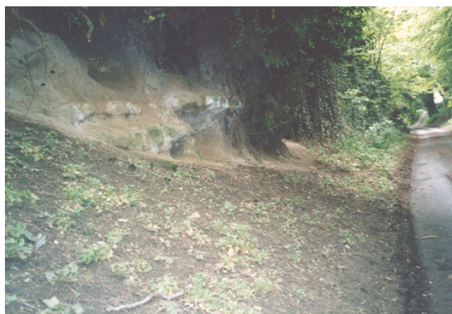
Photograph 1: Hartmoor Road - Doggers protrude from the bank sides showing the fragmented nature of the layer. The doggers support the rock above until sufficient erosion allows the individual blocks to fall out.
