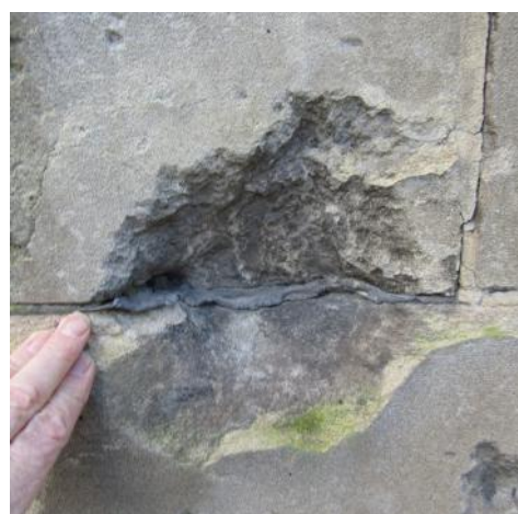
Fig. 7: Labour Exchange impact crater with deformation of the lead damp course
