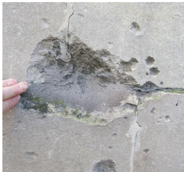
Fig. 6: Labour Exchange impact crater across 2 blocks where the boundary has been lost. Note the granular nature of the weathered surface of the limestone, contrasting with the finer-grained nature of the stone within the crater.
