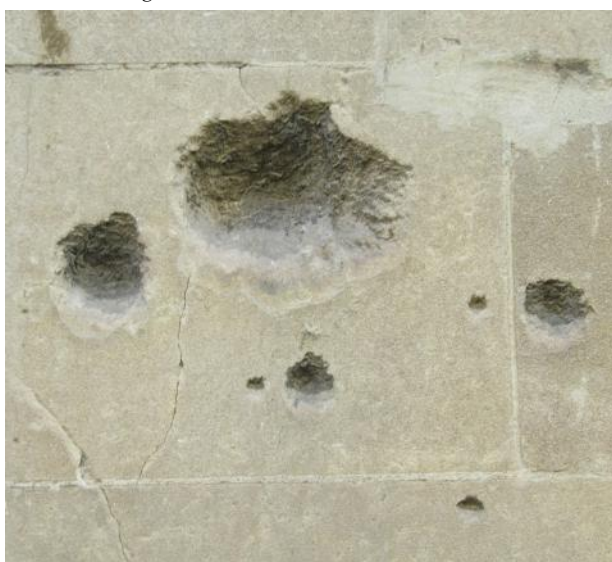
Fig. 4: Labour Exchange impact craters close-up with smooth interior compared with weathered stone.
