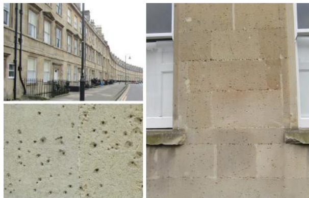
Fig. 12: The Paragon, a classic Georgian street in Bath, with an area of small impact holes, here many with a central hole, in some cases occupied by metal. Stone blocks 30 cm high.
