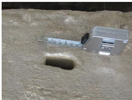
Fig. 6 A: An 18 th C bolt hole, length 5.5 cm, from a pediment from the Duke of Kingston's house, built c1750. Note the neat cut of the hole. Stone store, Roman Bath.
