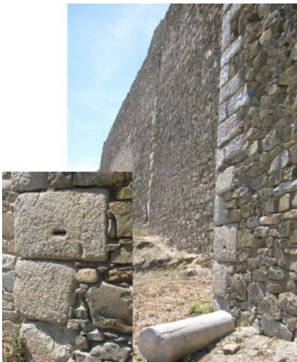
Fig. 2B: Bolt hole in granite block in wall of Roman fort (later rebuilt), Mertola, Portugal
