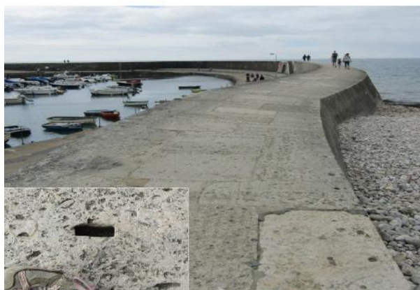
Fig. 6C: The Cobb, Lyme Regis composed of blocks of Portland Stone (mostly of the variety Roach), many with bolt holes.
