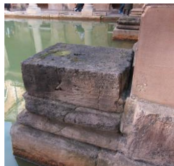
Fig. 3: The contrast between Roman (on the left, a column base) and late 19 th Century stone (upper right). A bolt hole on the top of the Roman stone is 11 cm in length. Great Bath, Bath.
