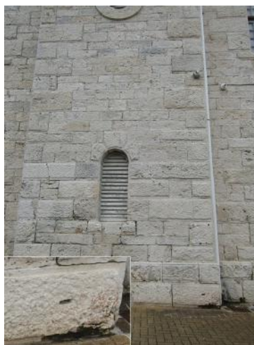
Fig. 6B: Bolt hole in a block of Pleistocene limestone at the base of the Royal Naval Clocktower, Bermuda
